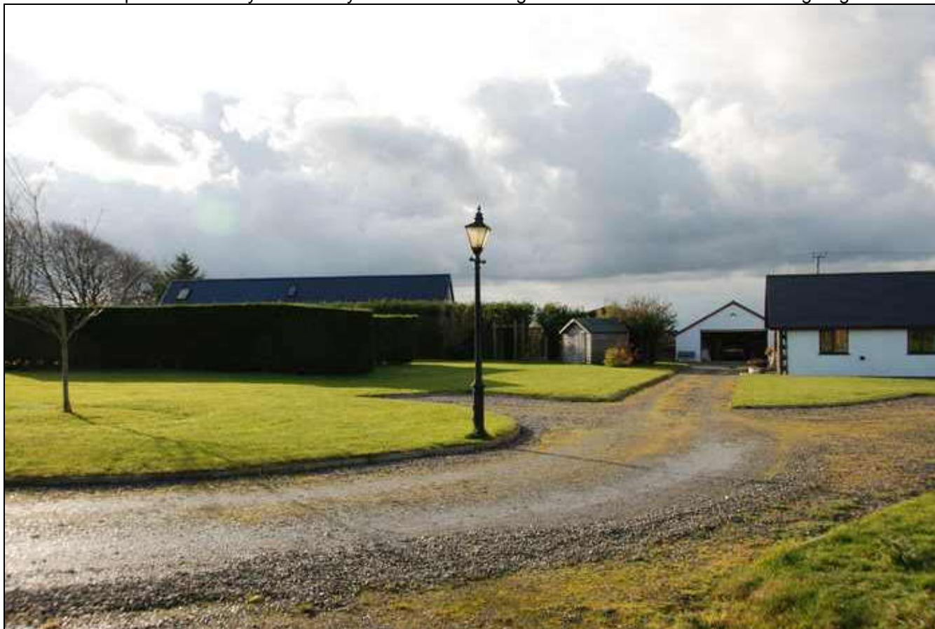
A separate driveway leads away from the outbuilding area round to the residence and garage
